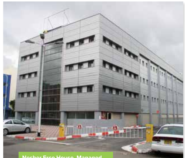
Nesher Erco House, Managed and Maintained by Natam
